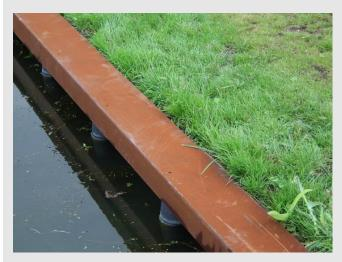
The characteristic rust colour of CorTen steel gives the sheet pile a modern look. A deck apron made of CorTen steel has a technical lifespan of 50 years.
